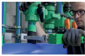
1. The aquatherm component unit is welded on the media pipe using special saddle welding tools.
