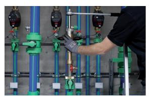
3. The drilling is carried out by actuating the manual ratchet and careful feed via the ball handles.
